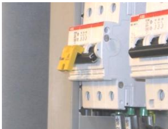
Fig. 2: The device blocks the circuit breaker open position
