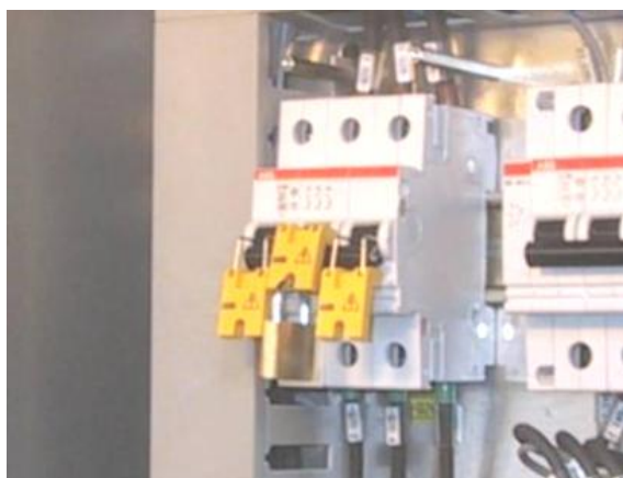
Fig. 2: Every pole of the circuit breaker is padlocked
