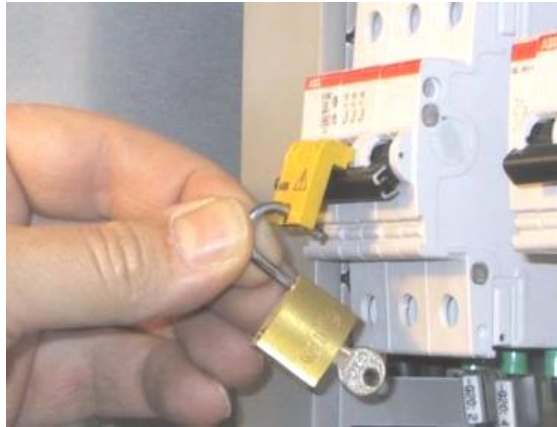
Fig. 3: First padlock inserted
