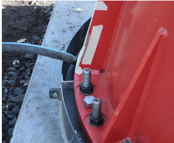
Figure 2: grouting of the telescope Base
