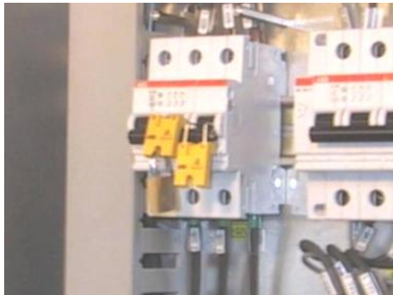
Fig. 1: A second locking device is inserted
