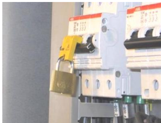
Fig. 4: First padlock blocked
