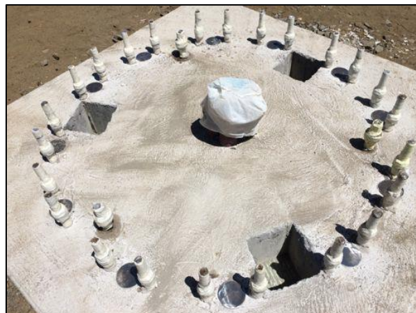
Figure 11. Anchors bolts emerging from the foundations of the ASTRI-Horn prototype
