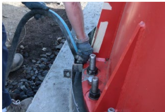
Grouting the Mechanical foundation interface
