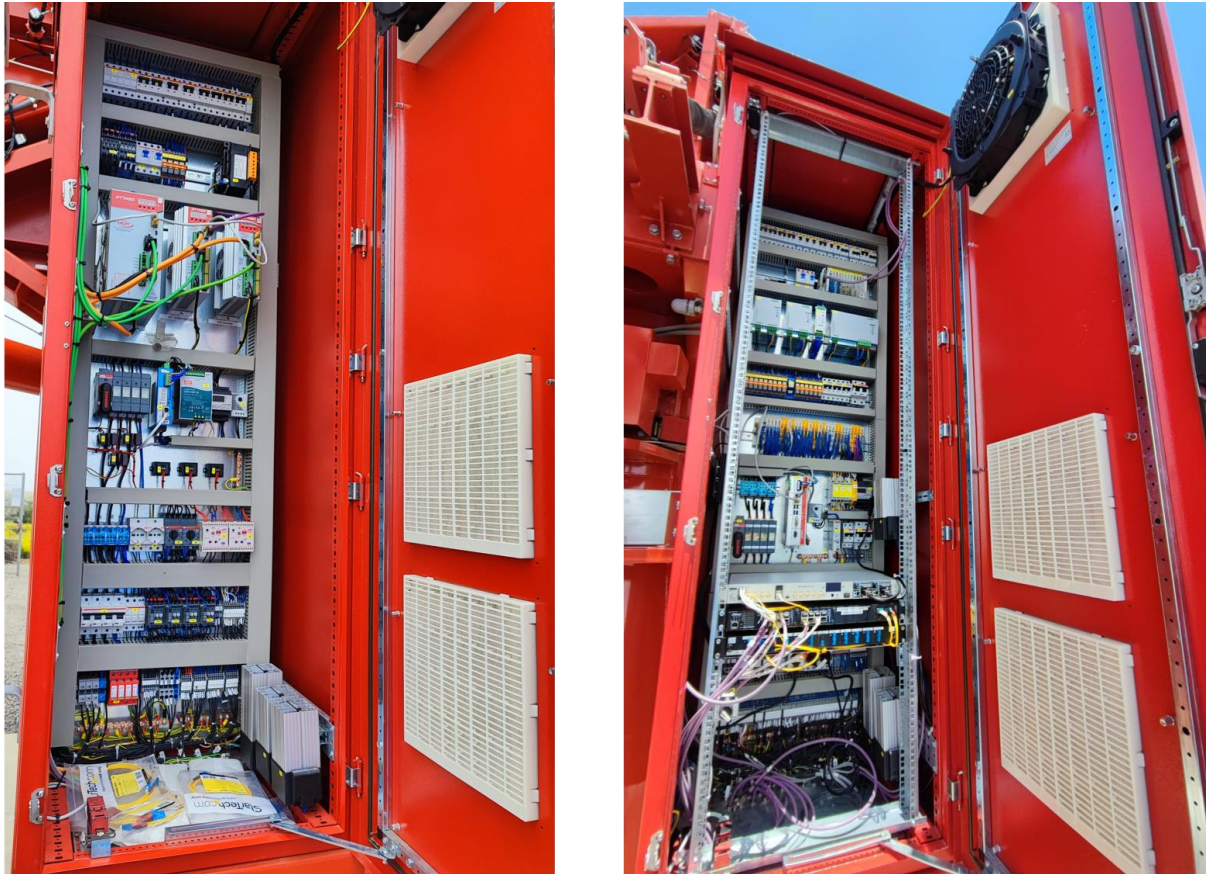
Figure 7. On the left the ASTRI Mini-Array Telescope Power Cabinet and on the right ASTRI Mini-Array Telescope Control Cabinet.
