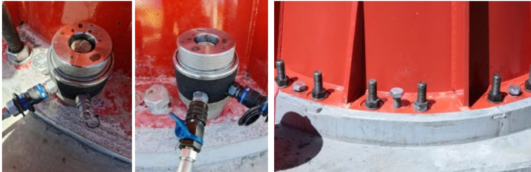
Anchor preloading
