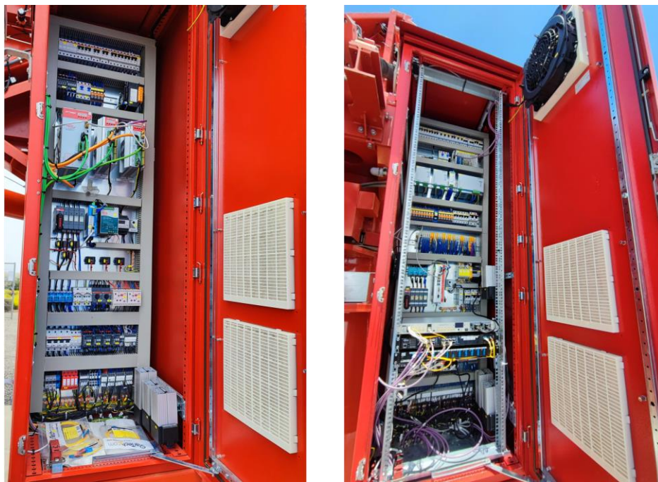
Figure 4-4: the figure shows: on the left the ASTRI Mini-Array Telescope Power Cabinet and on the right the ASTRI Mini-Array Telescope Control Cabinet.
